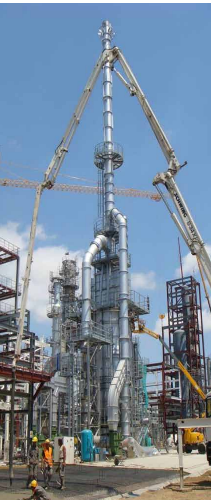
Lukoil Refinery, Burgas Bulgaria
