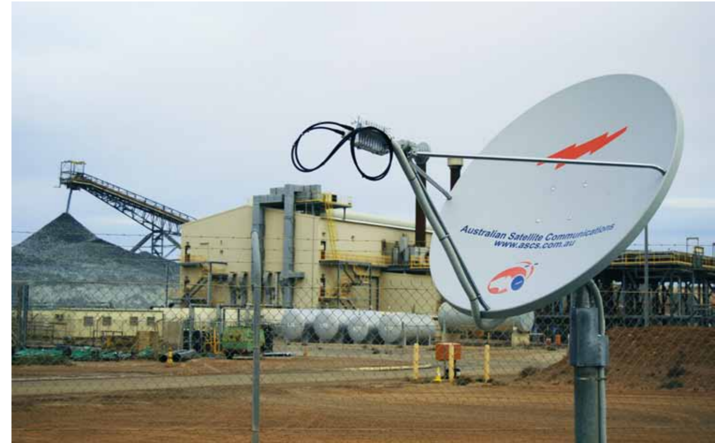
Remote site communication
