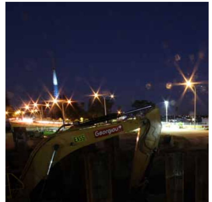
Early works on the main drain
