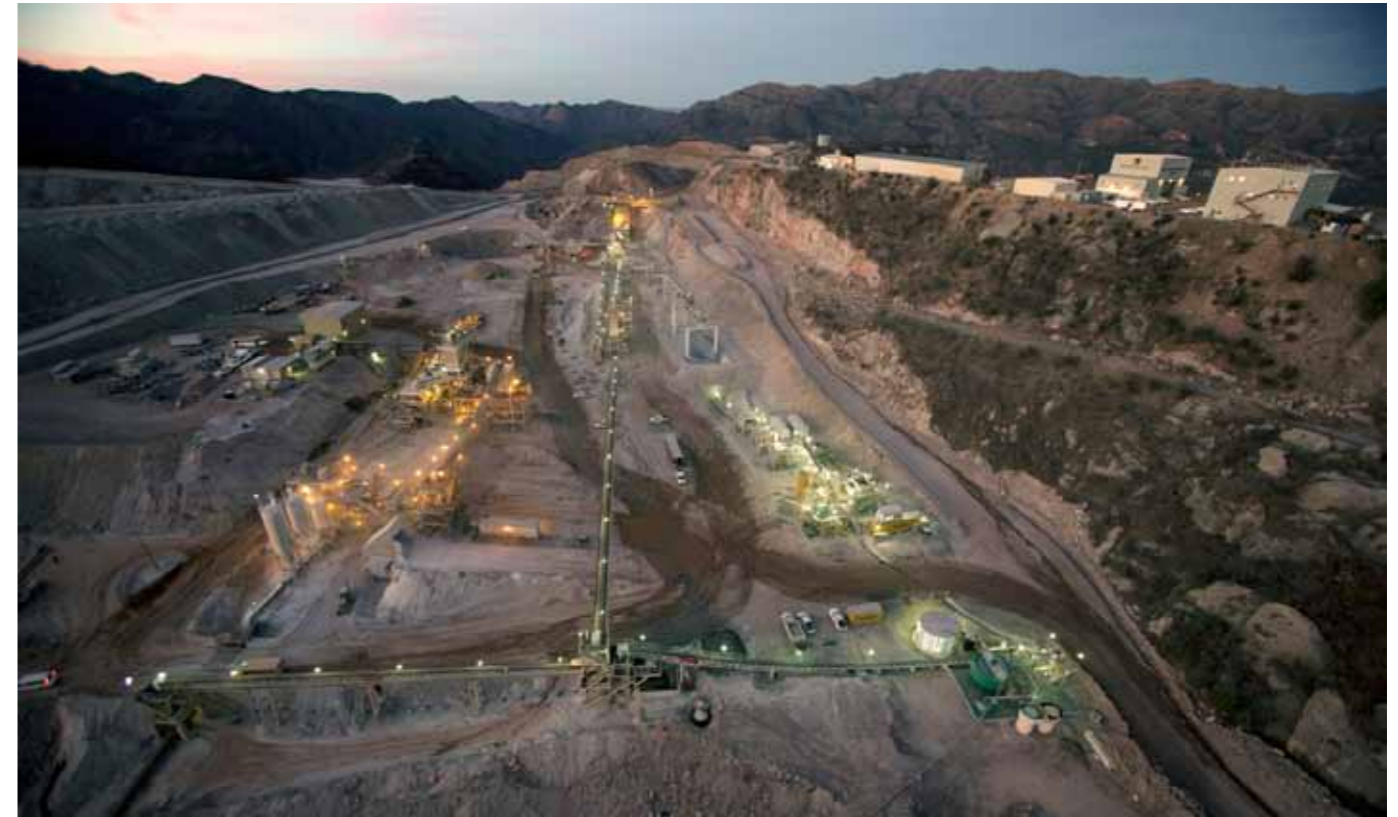
Overview of Mulatos crushing circuit
