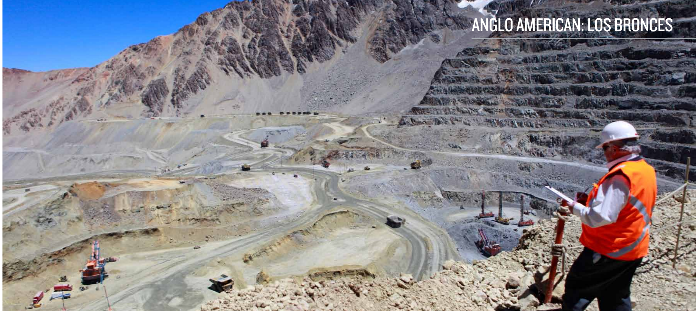
General view of the open pit at Los Bronces
