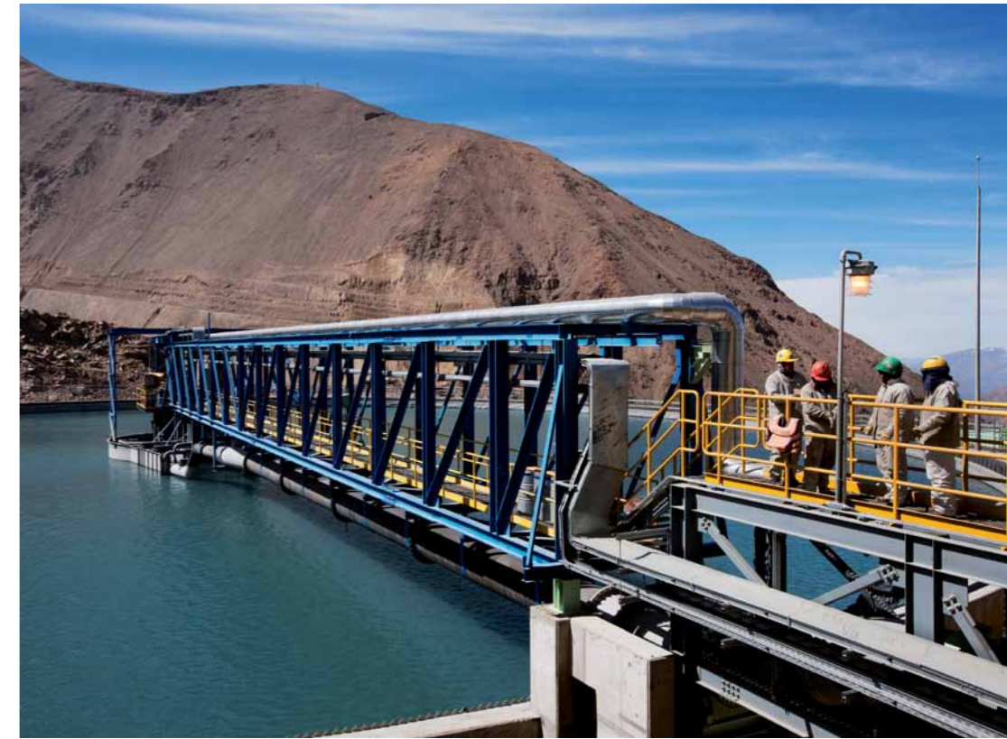
Pulp thickener at Los Bronces, Confluencia facility
