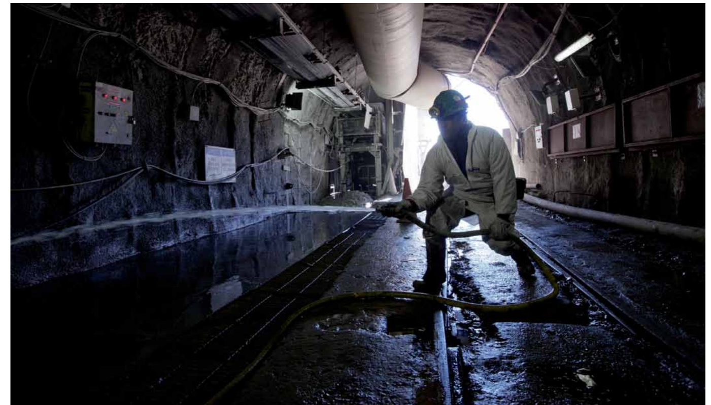
Routine cleanup of the exploration access tunnel
