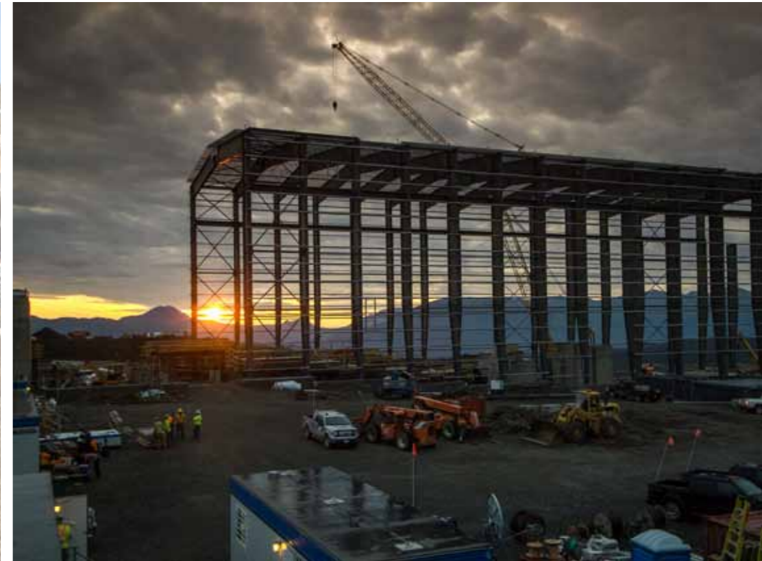
Red Chris mine construction site. Photo provided by Imperial Metals Corporation
