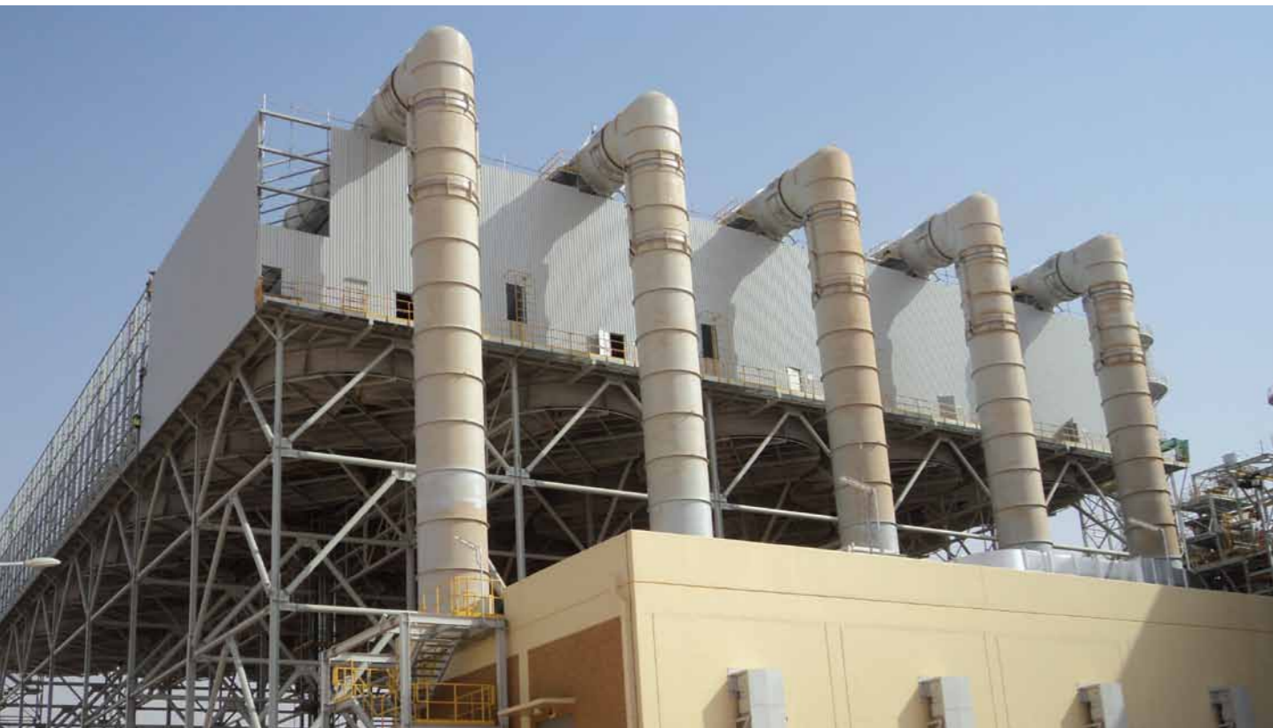
Block 2 air cooled condenser with associated steam feed pipes
