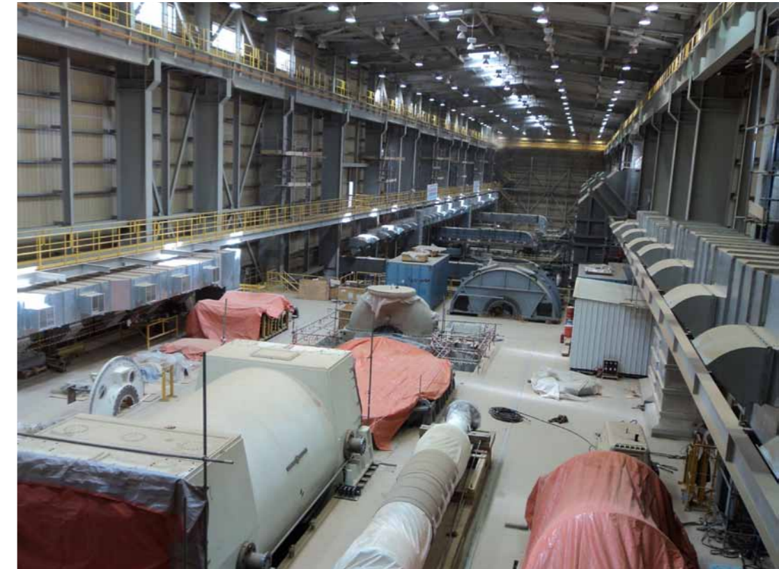
Block 2 turbine hall showing the steam turbine generator under erection
