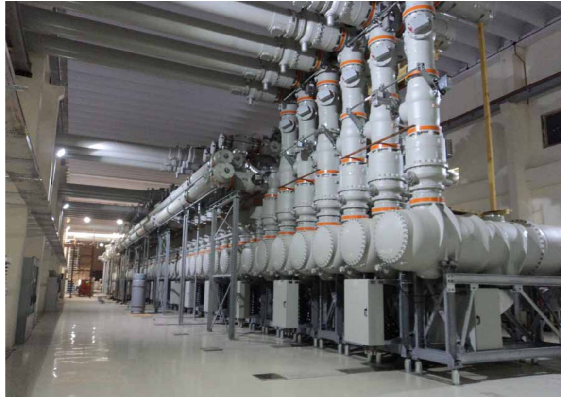
Phase I of the Gas Insulated Substation (GIS) under erection
