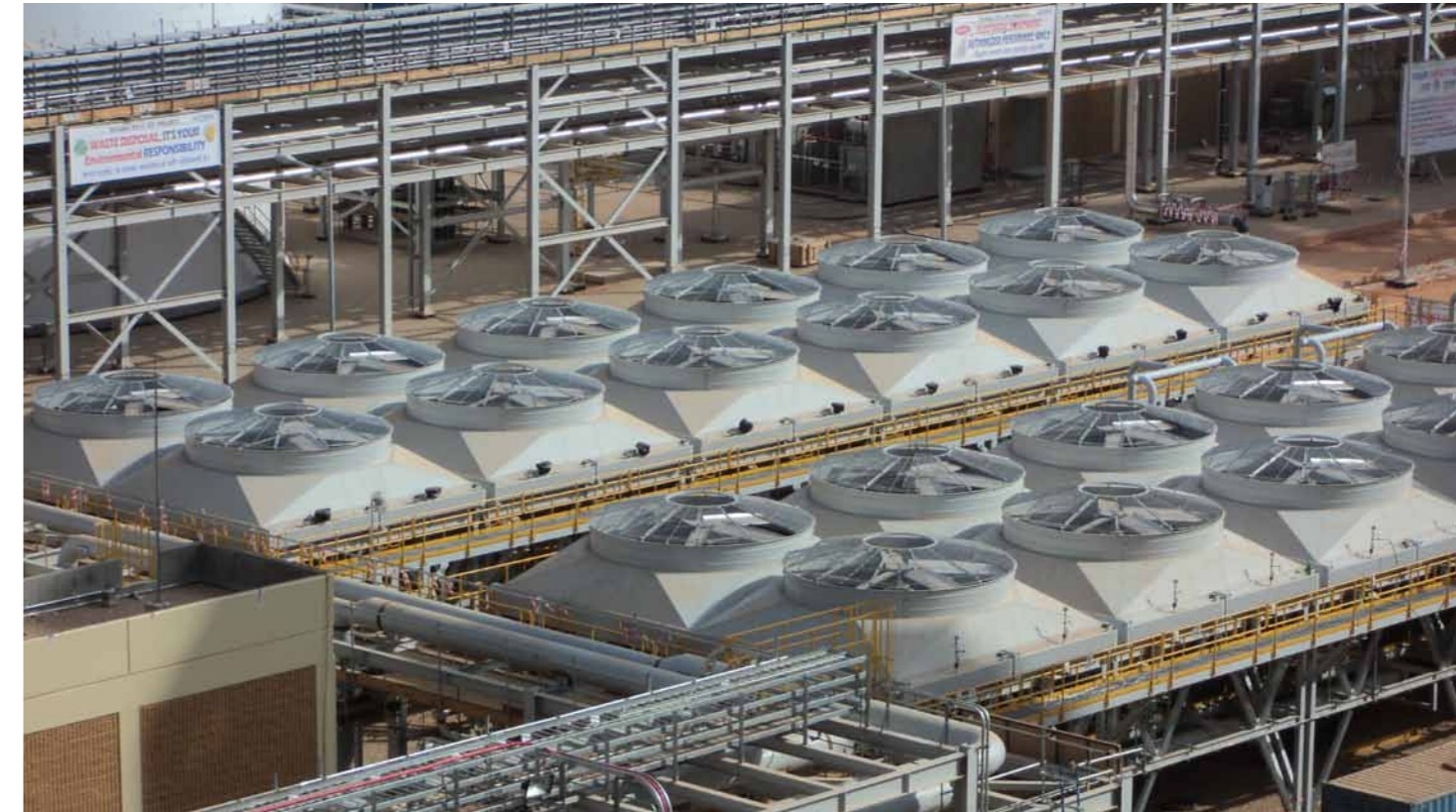
Coolers for the closed cooling water system on Block 2
