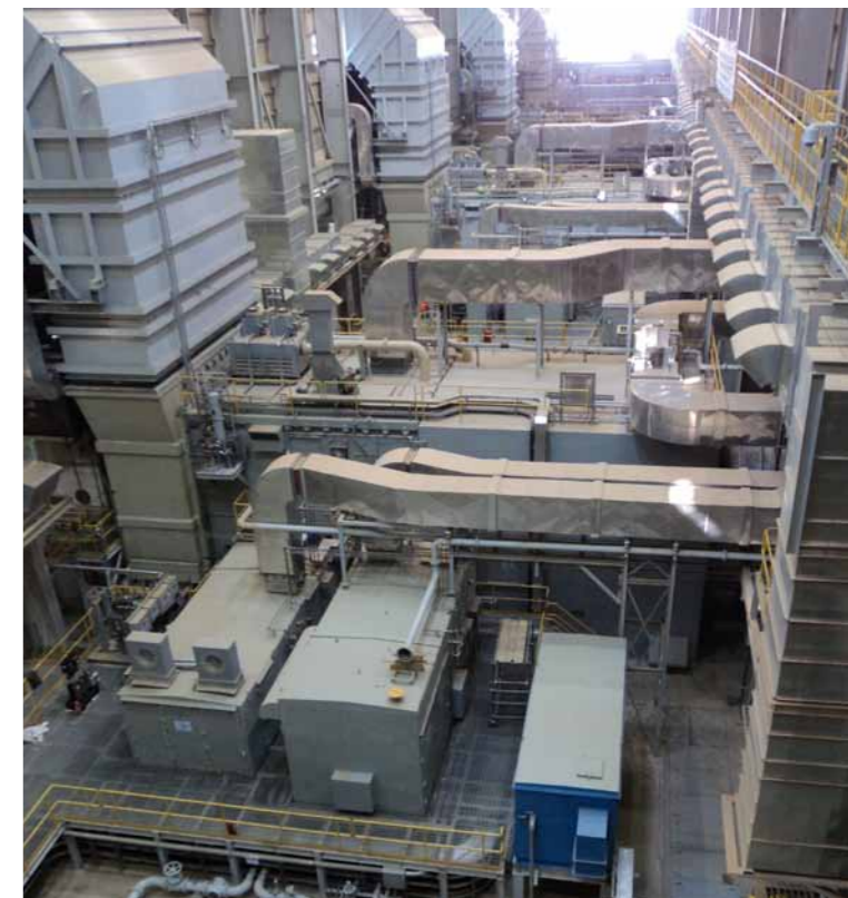
Block I turbine hall prior to the successful first fire of GTII
