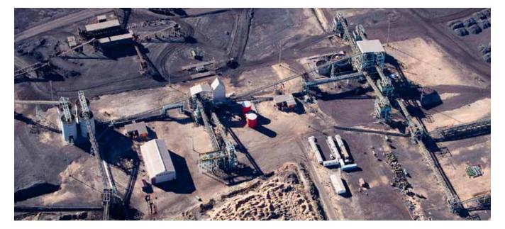
purpose-built silos, each with a capacity of 2,000 tonnes. "While the beneficiation plant is on the same site as the Nchwaning mine, these silos act as a fail-safe mechanism," explains Letaba. "Should something go wrong underground and we are unable to bring the ore to the surface, we do not have to shut down the plant as we still have 8,000 tonnes to work with."
