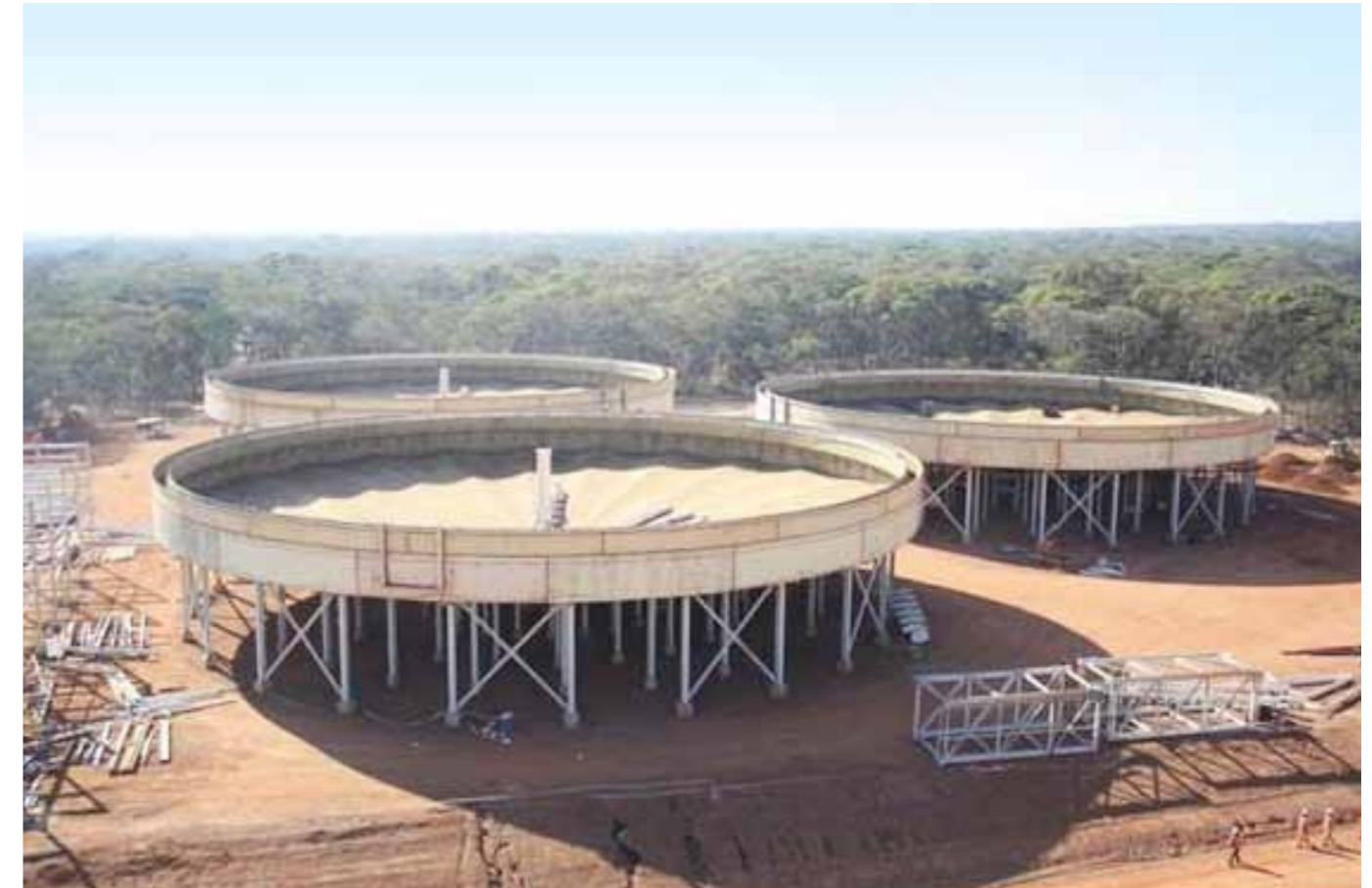
50m diameter tails thickeners
