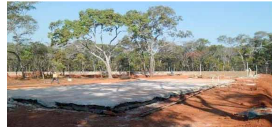
Trust school foundations laid
