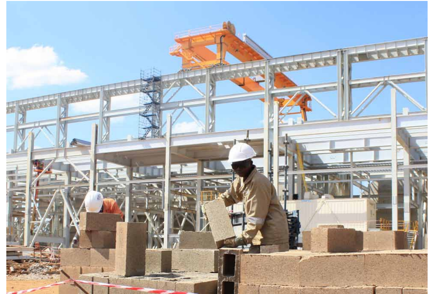
Process plant construction team
