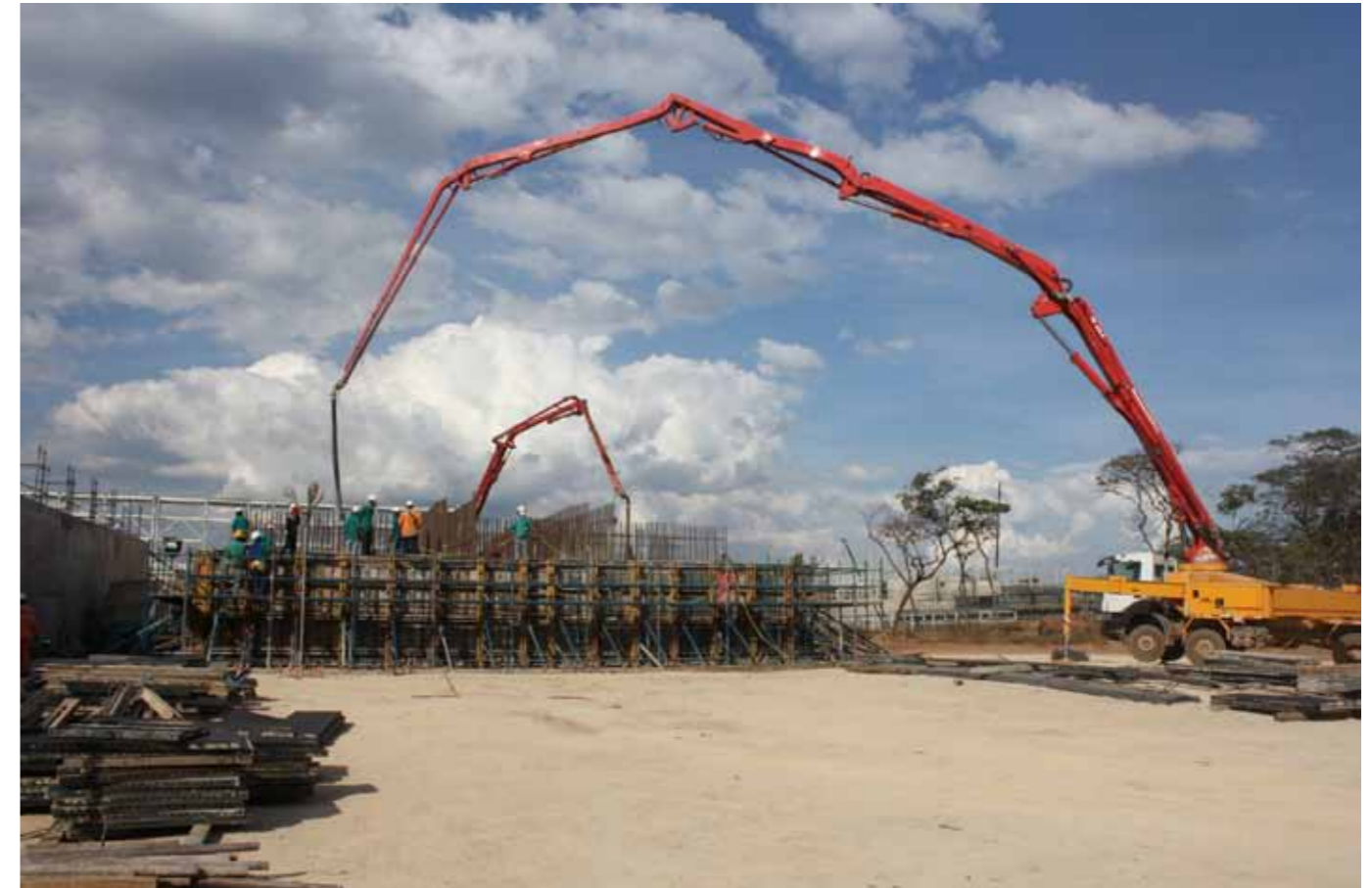
Stockpile pylon concrete placement
