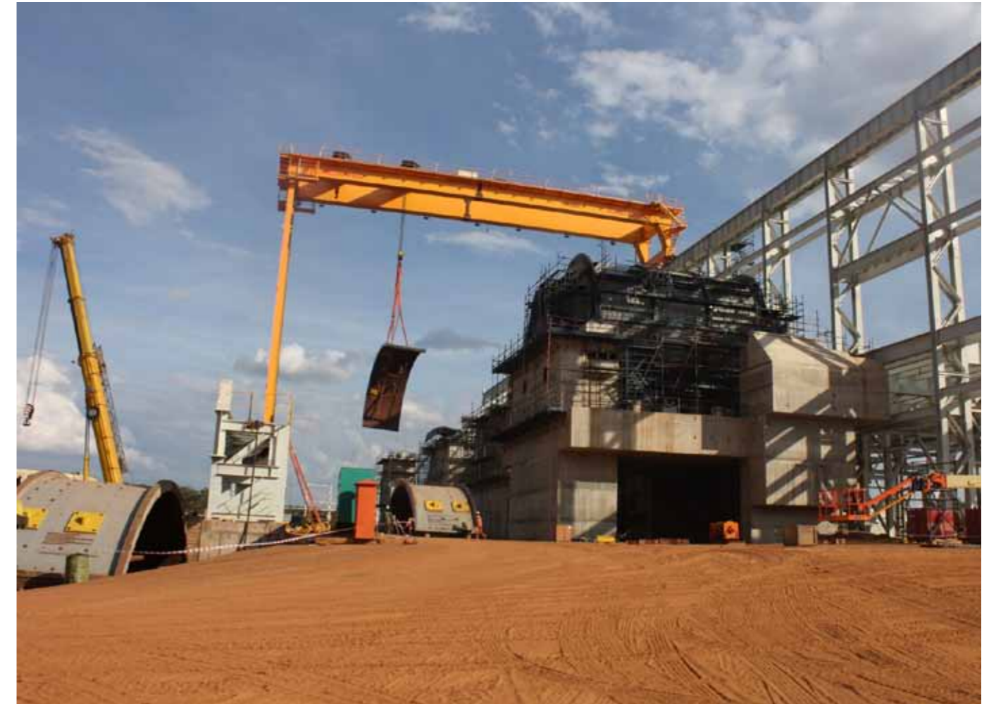
Mill area progress - second shell section being lifted into position
