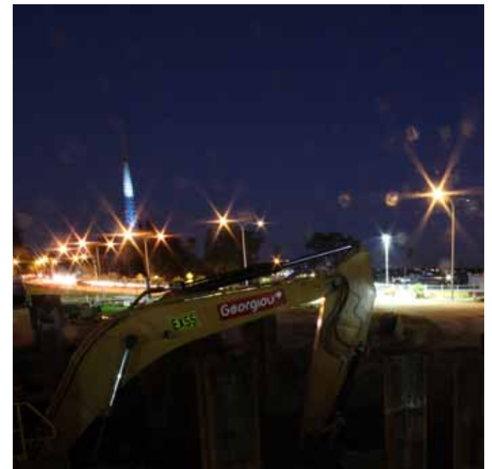
Early works on the main drain
