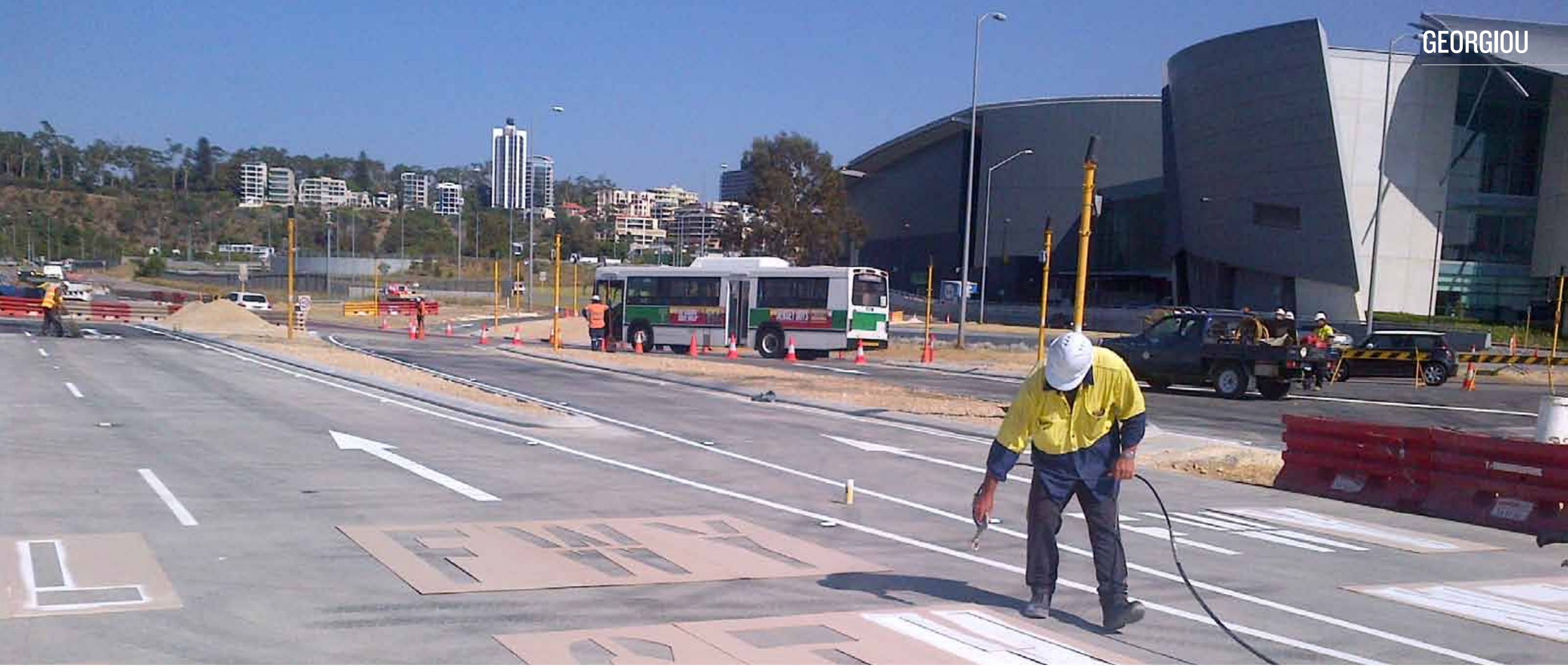
Linemarker preparing major road diversion
