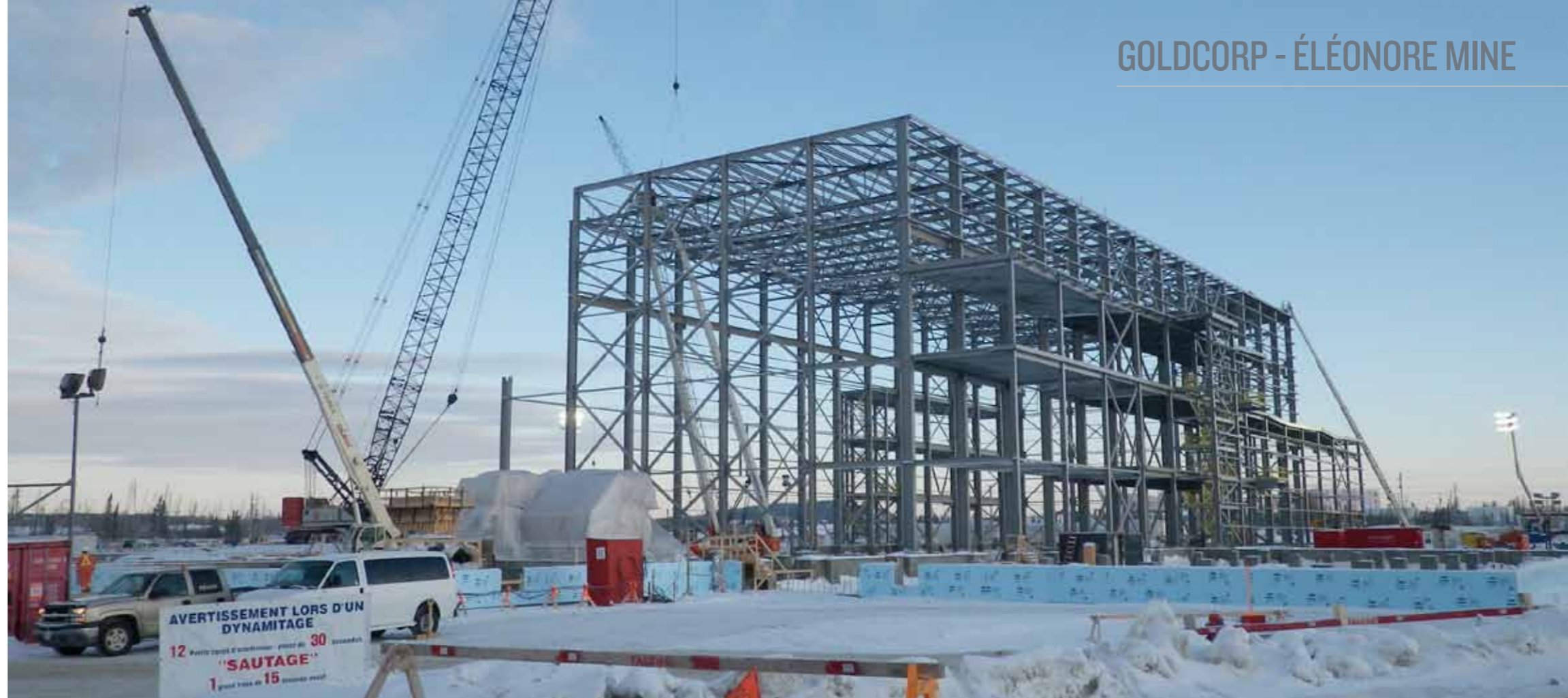
Concentrator under construction
