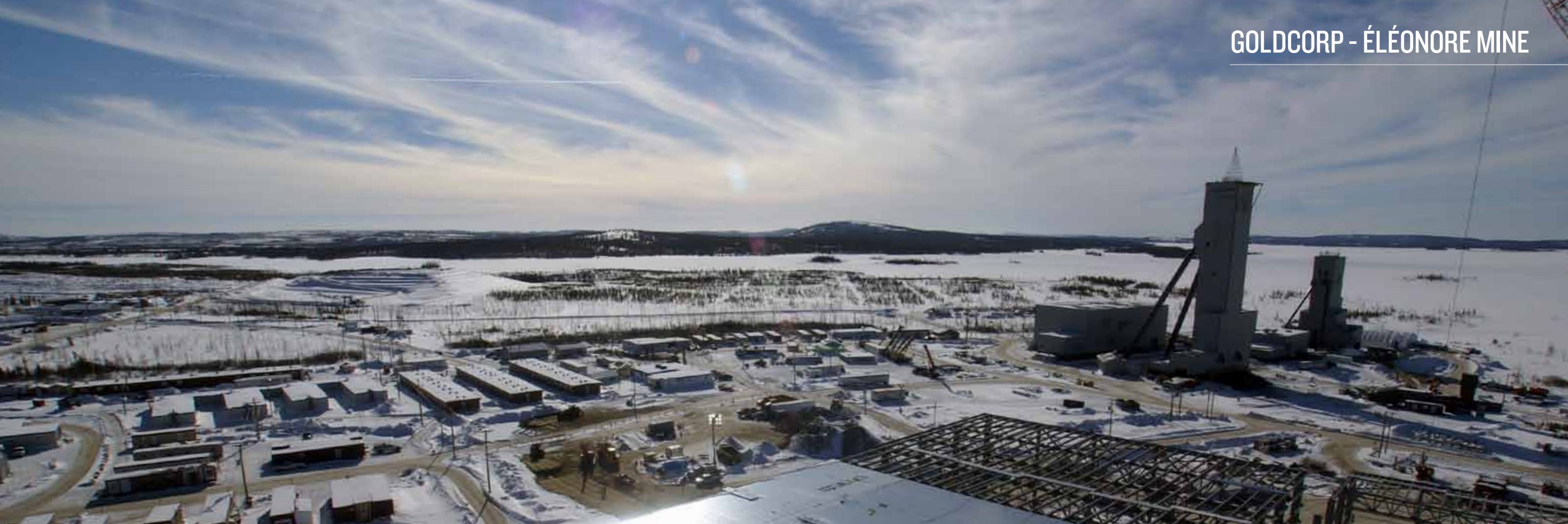
Aerial view of the operations
