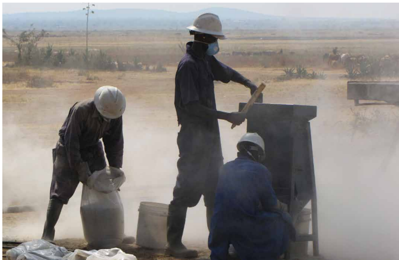
Local contractors are used wherever possible
