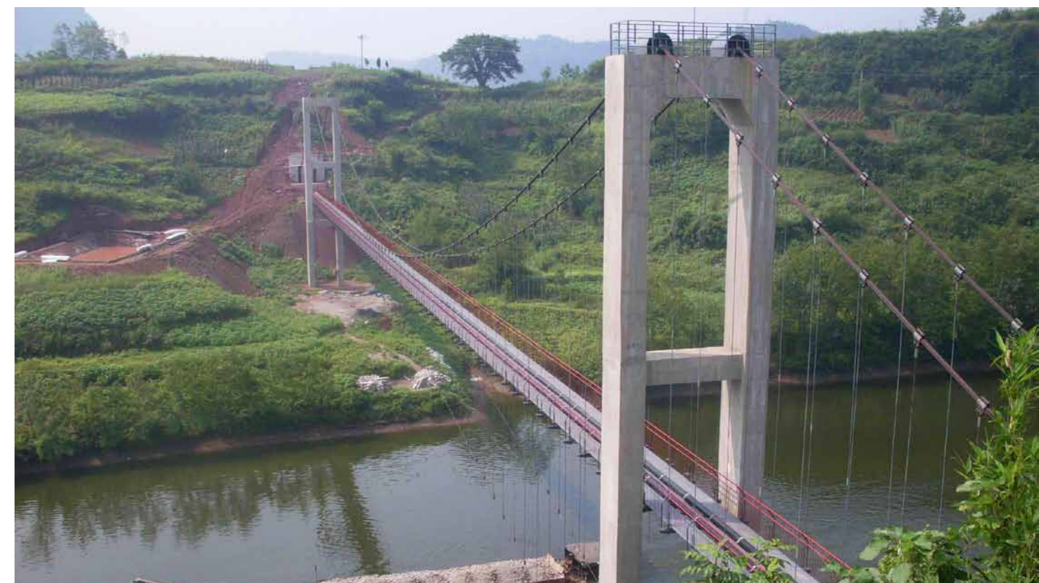
Phosphorous acid pipeline
