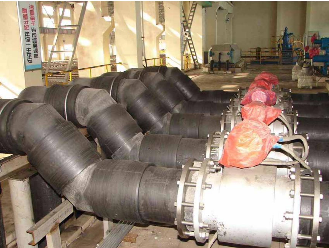
Sulfuric acid pipeline for copper mining
