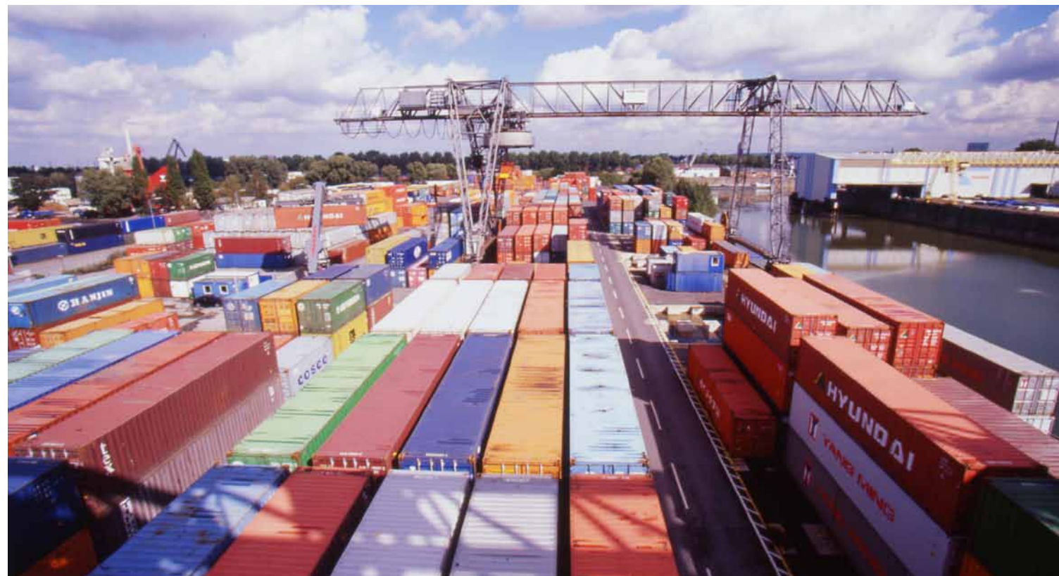
neska intermodal terminal
