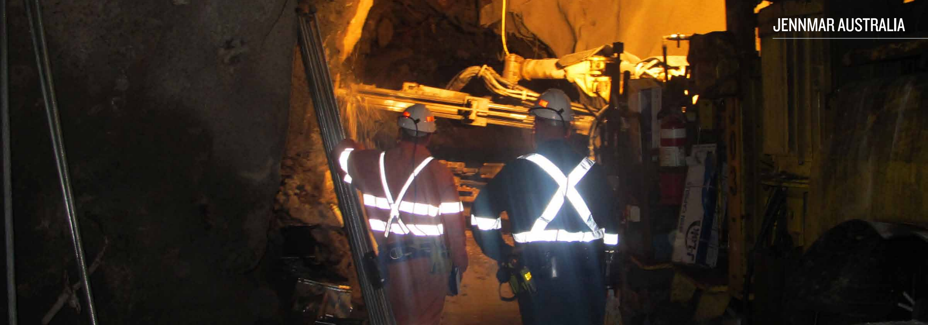
Workers underground during Yield Lok trials
