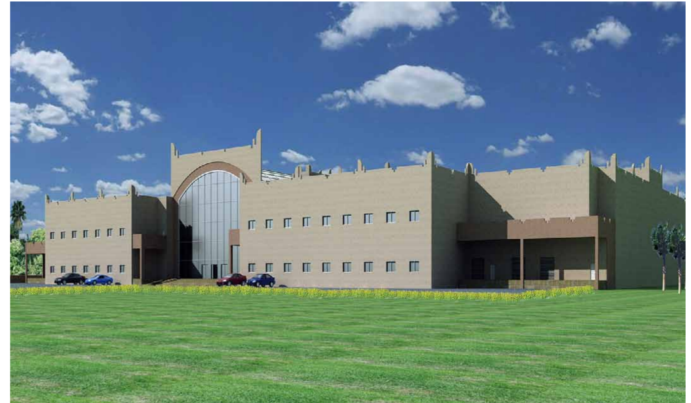
Julphar Insulin Plant
