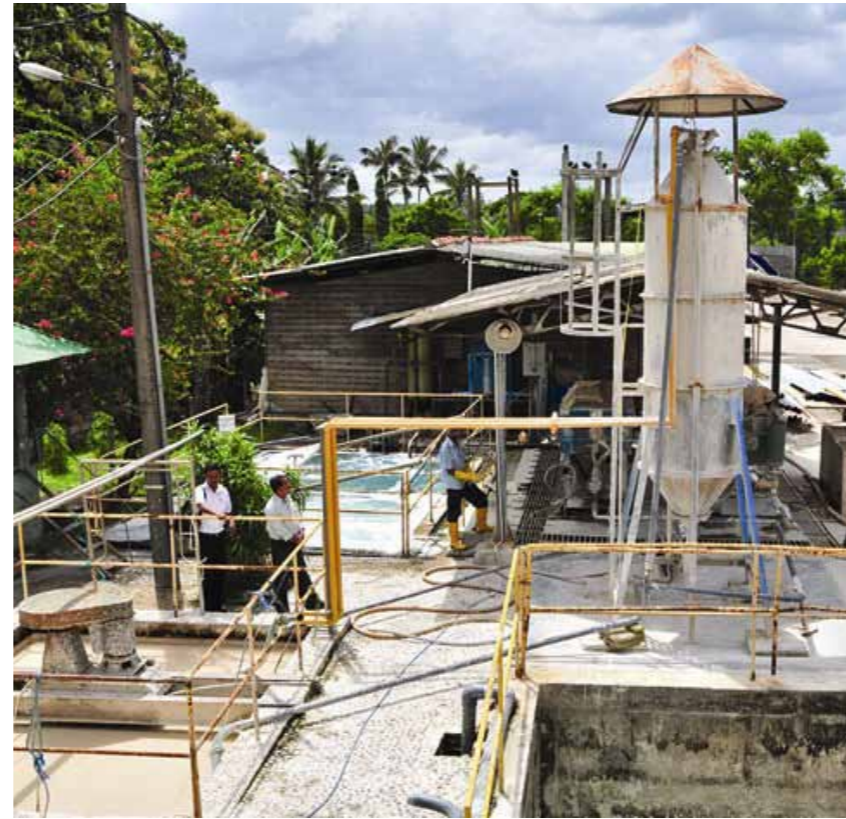
Effluent treatment plant
