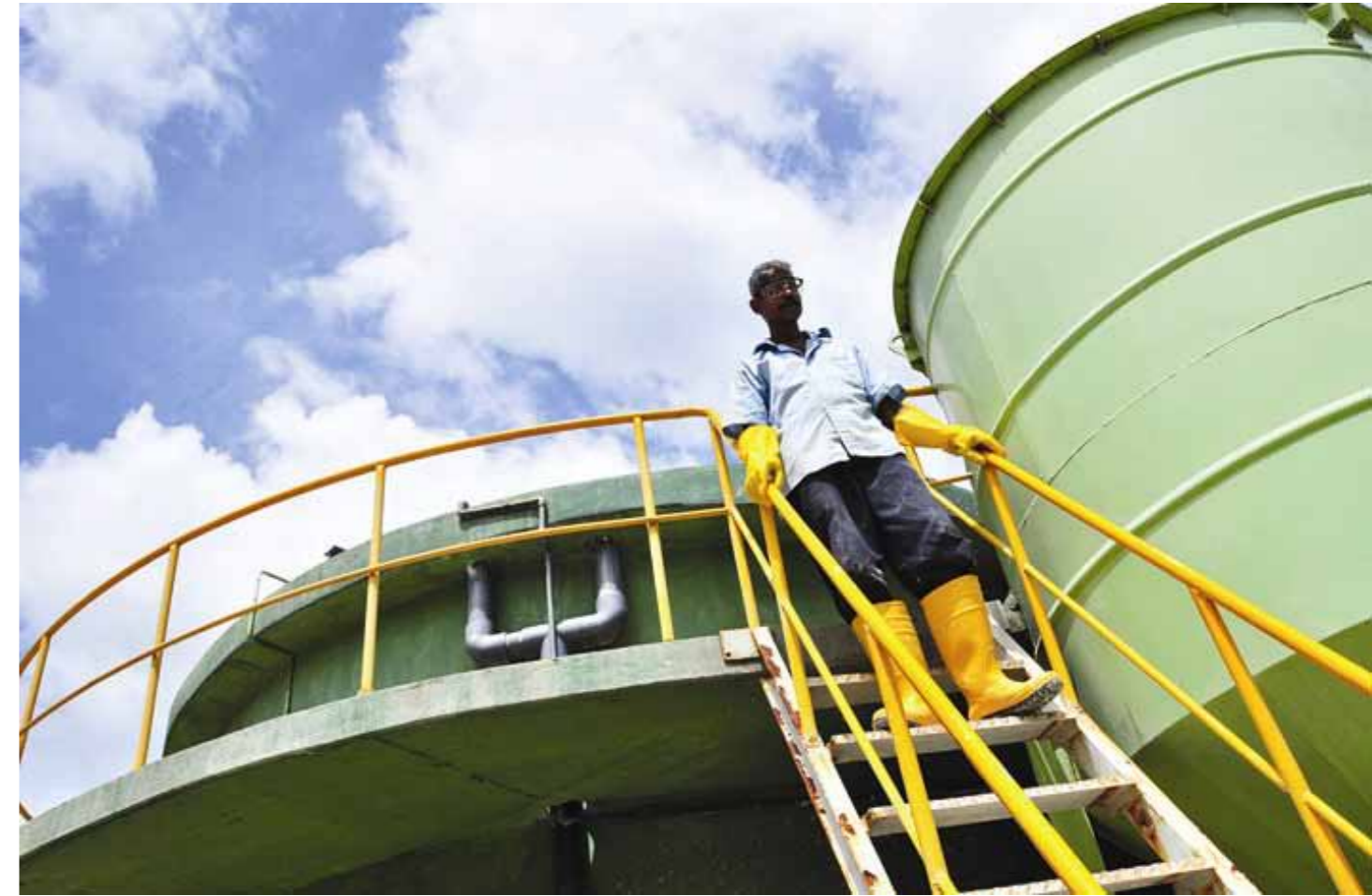
Effluent treatment plant
