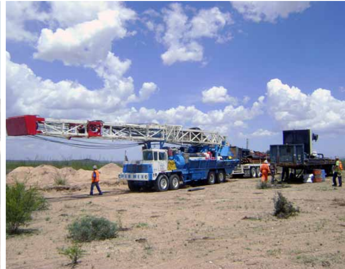
Commercial water well drilling rig for high velocity wells
