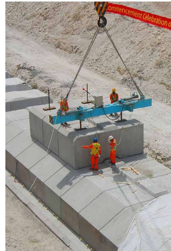
First quay wall block installed
