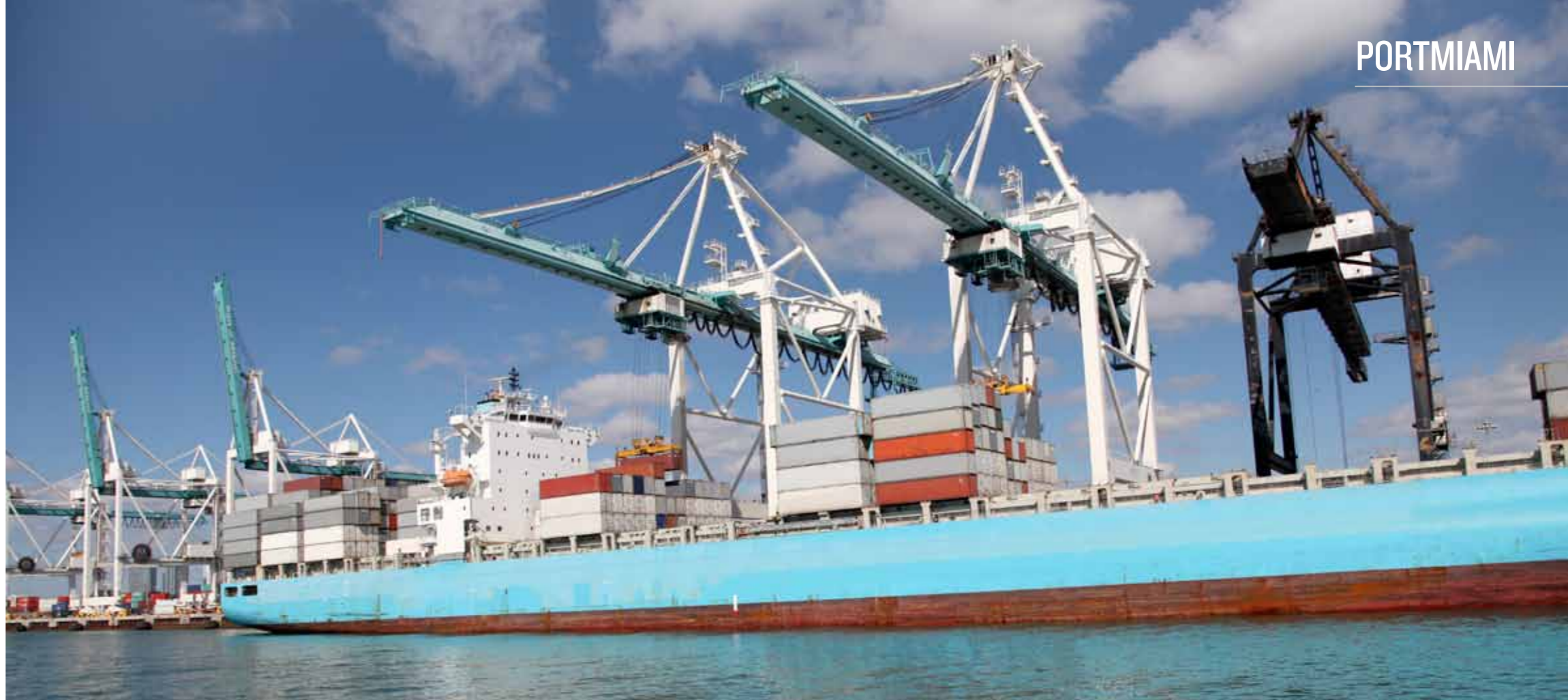
Cranes and container terminal
