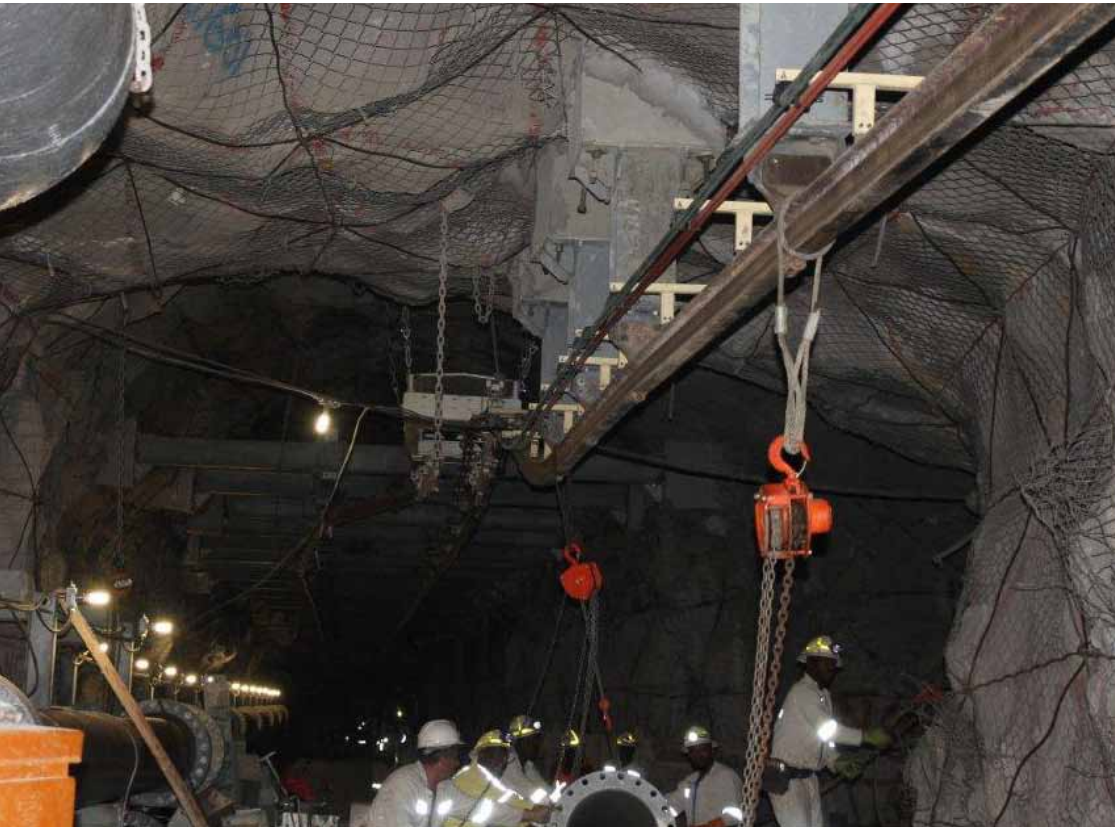
EMTS moves supplies and consumables underground
