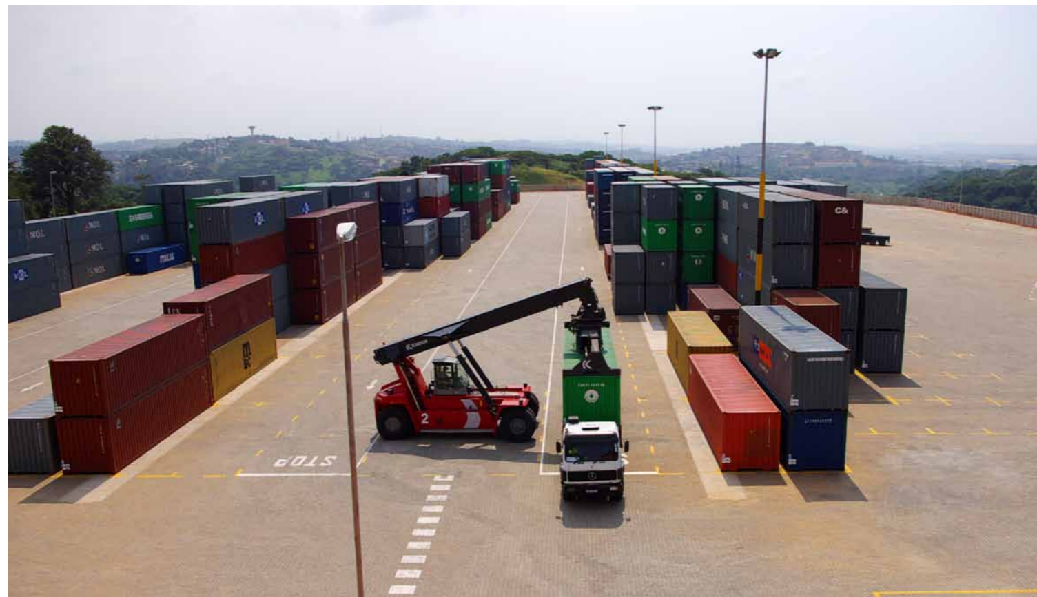
Container terminal in operation
