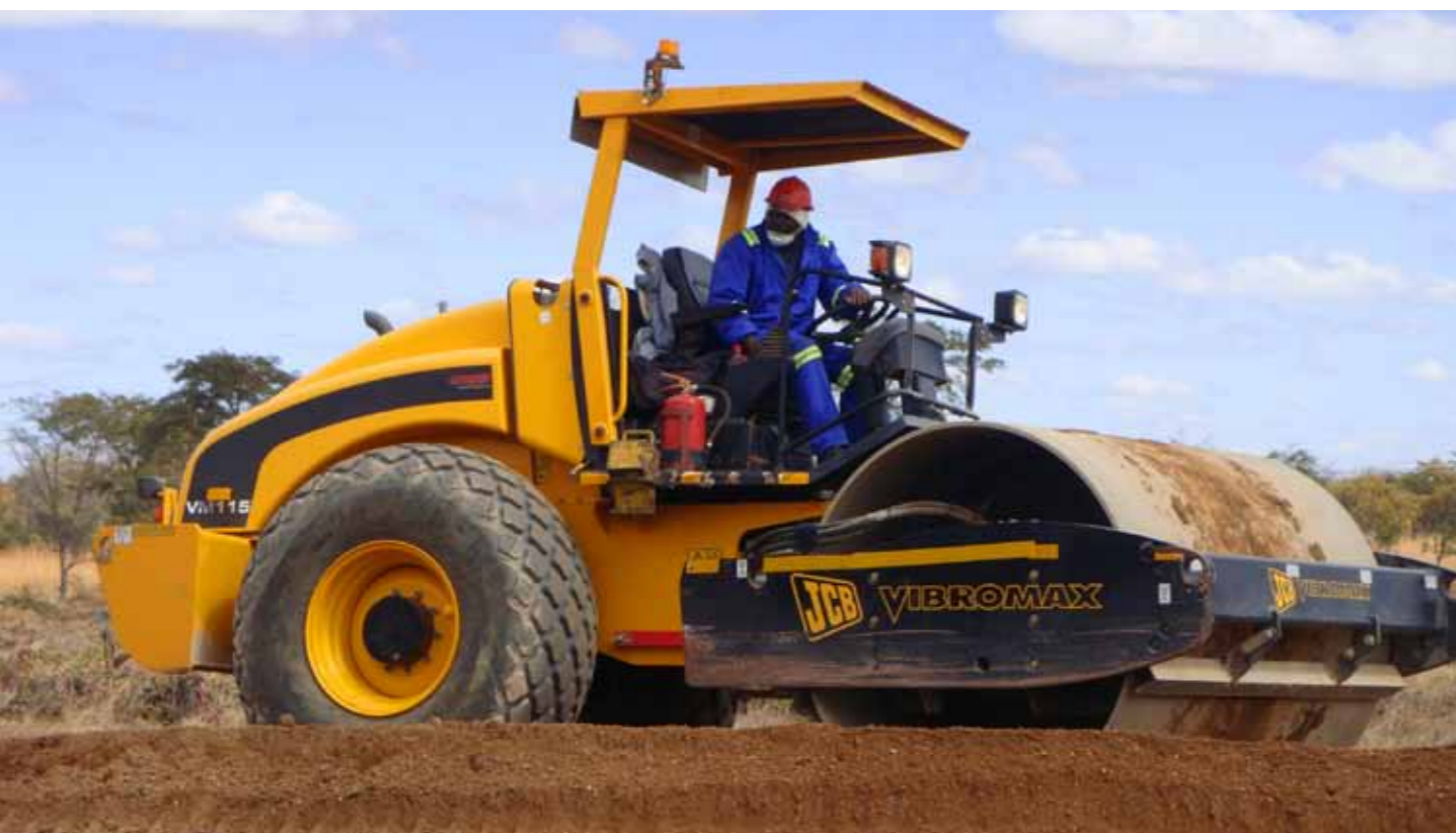
Vibrator at work
