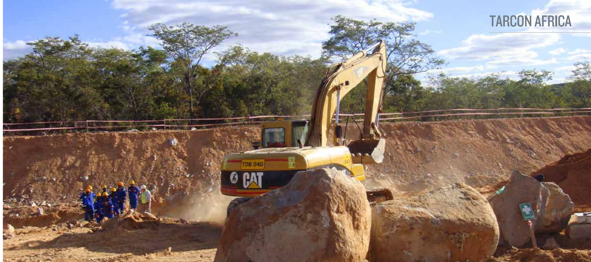
Island dam core trench excavation
