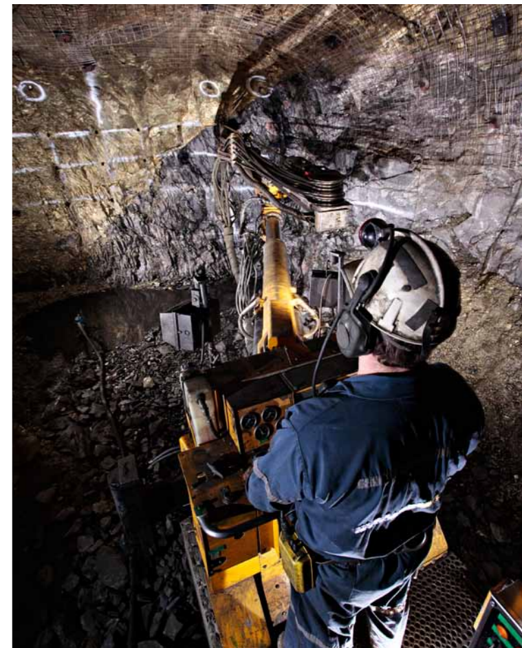
Jumbo driller at Coleman Mine
