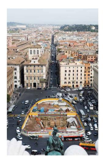
Grasping the context that Mr. Sciotti refers to is crucial to understanding the specific nature of the Linc C project. He tells us: "The soil of Rome is characterized by fluviallacustrine recent sediments with extreme vertical and lateral lithological variations, and gradual or abrupt transitions." In layman's terms, this means that Rome's soil has huge inconsistencies, creating obvious headaches for engineers involved in the construction of a metro line.
