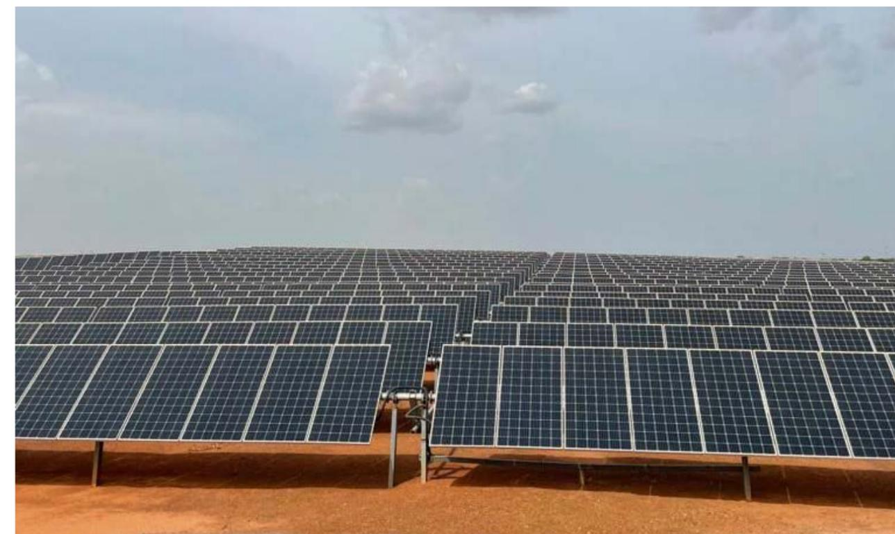
Loulo-Goukoto was chosen to pioneer an innovative solar power project, adding 20MW to the complex's grid, reducing the unit cost of its power, and cutting carbon emissions by around 40,000 tonnes per year
